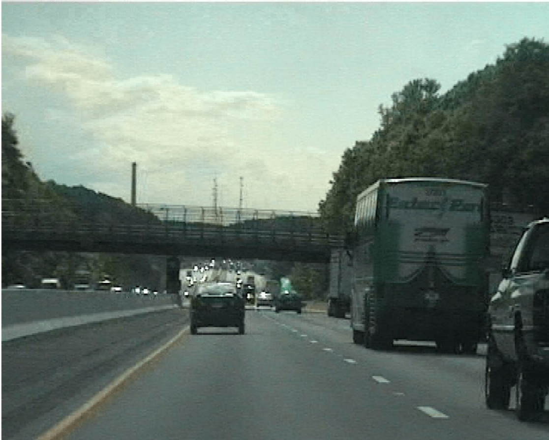
Image after deinterlacing
